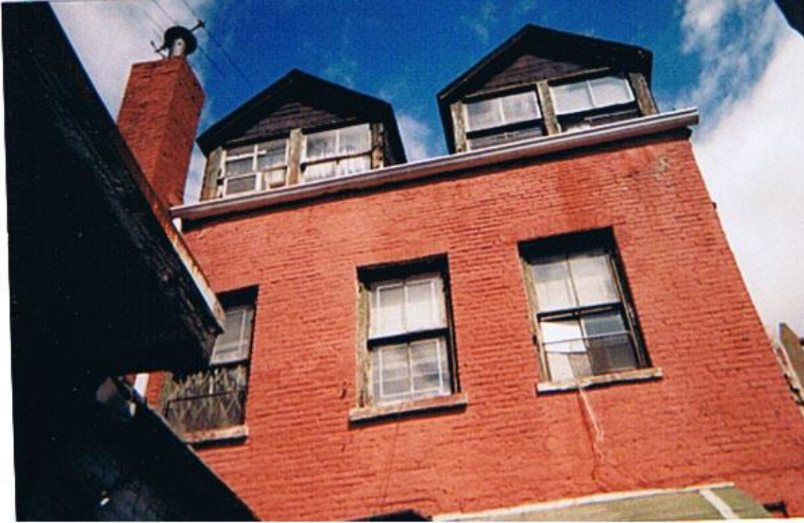
Rear photo 120 South 8 th Street
